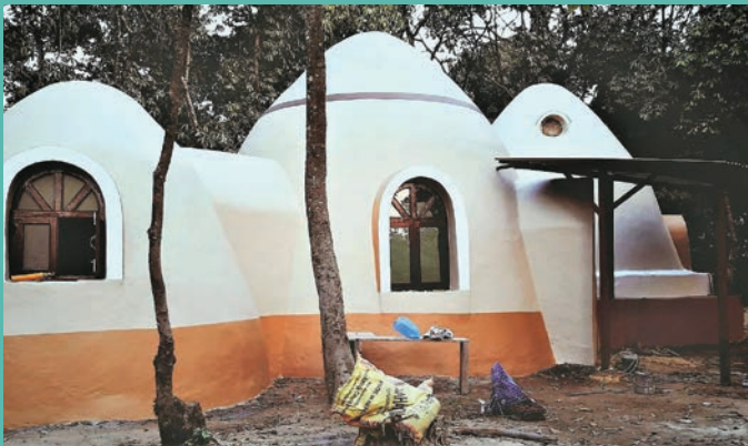
A unique "dome home" is among the Earthbag building projects LaSota has overseen.
