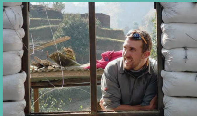
Daniel LaSota, '09, peers through the window of an in-progress building.
