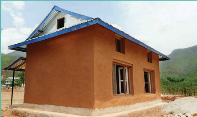
A completed Earthbag home with traditional adobe plaster.
