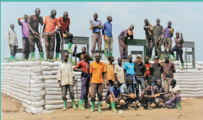
In Uganda, LaSota helps locals build the nation's first Earthbag school.
